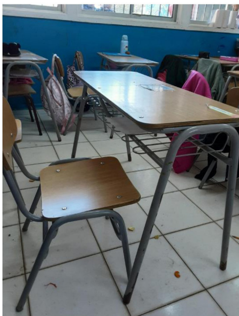
Figure 2. Ceramic Tile Flooring and Classroom Furniture Without Protective Rubber Feet.
